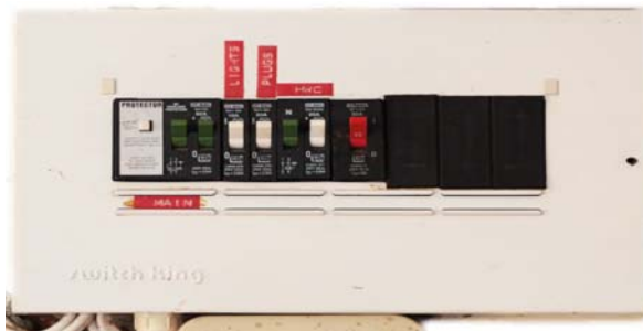
An electrical distribution board with circuit breakers
