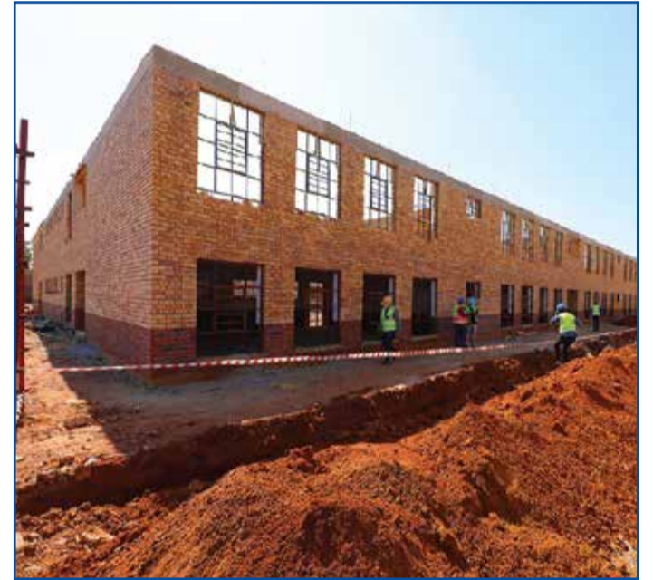
Newly built classrooms with concrete slabs
