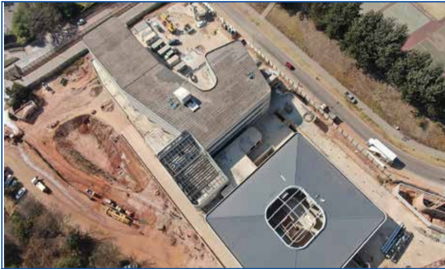
Pathology Unit Aerial View
