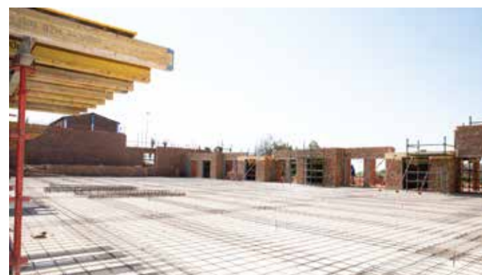
Refithlile Pele construction site
