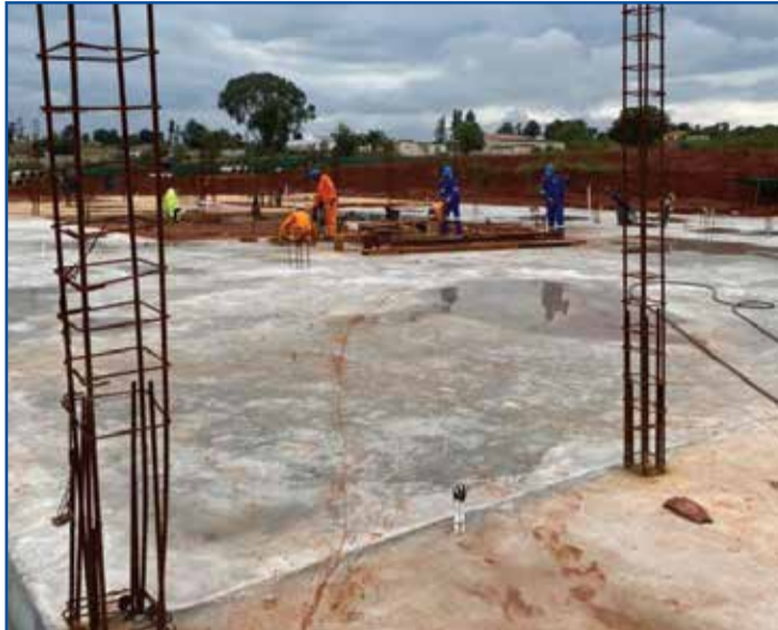
Contractors at work sites (above), & SMMEs at registration centres (right)
