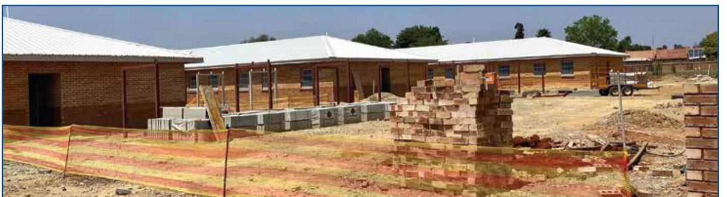
Newly built WK Du Plessis classrooms and facilities
