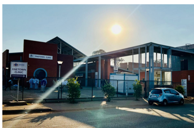
Accelerated delivery and refurbishments of our infrastructure
